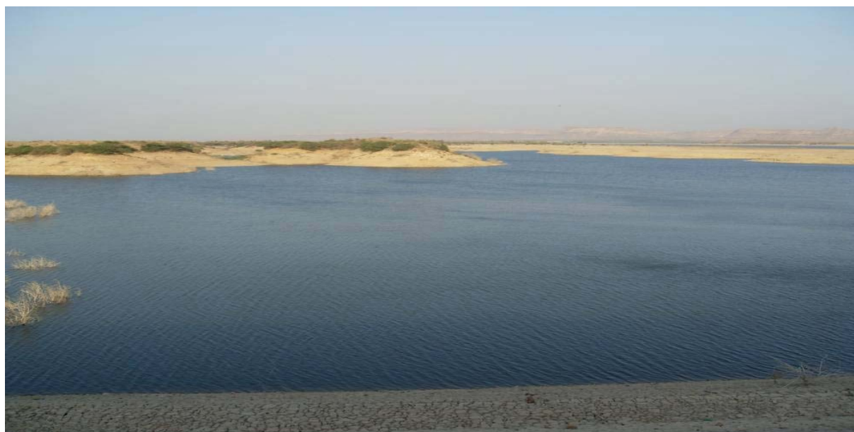
Fig. 3. View of Hub Dam.
